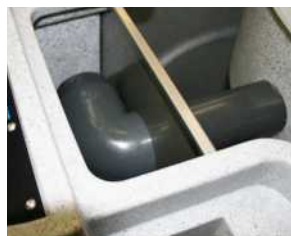
Figure 17.3 - By-pass in operation
